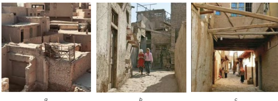
Fig. 5. Stilted Residential Houses
